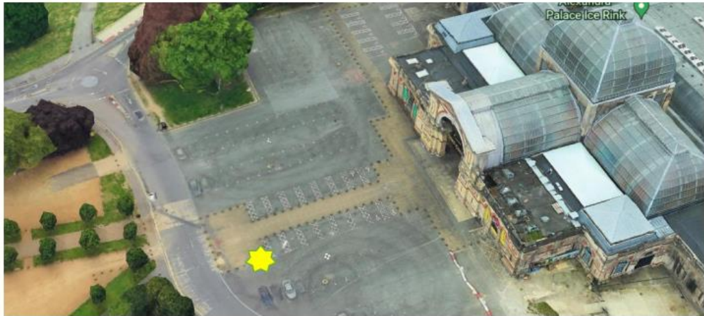
East car park – 3no pay terminals
